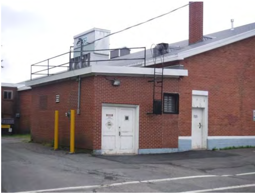
M1: Refrigeration Plant view from the street. Evaporator located on Roof
