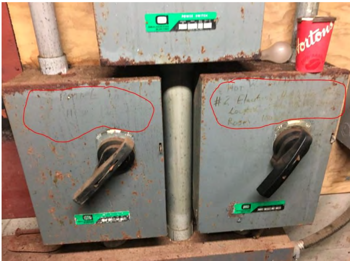
E10: Disconnect Switches labeled with Sharpie. No Electrical shock or arc flash warnings
