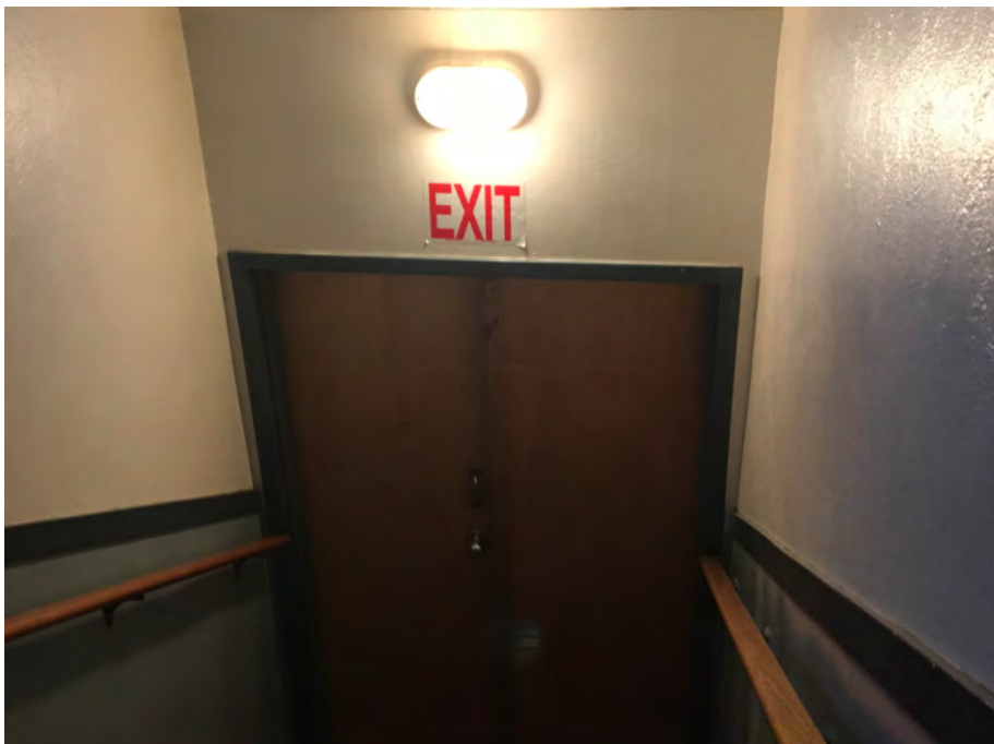
E19: No emergency lighting at mezzanine exit
