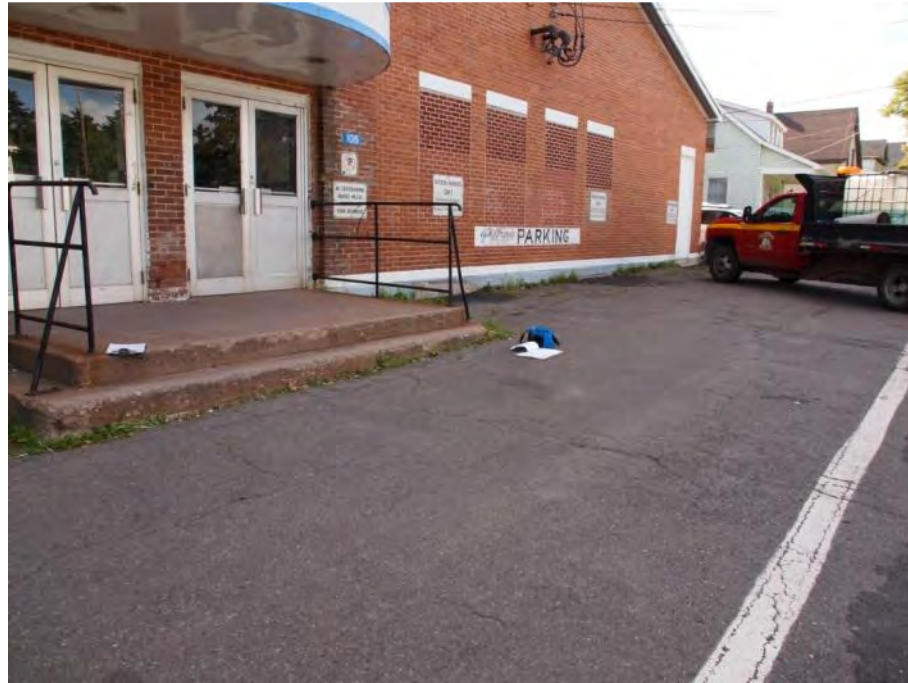
A1: Under linedated Parking near main entrance
