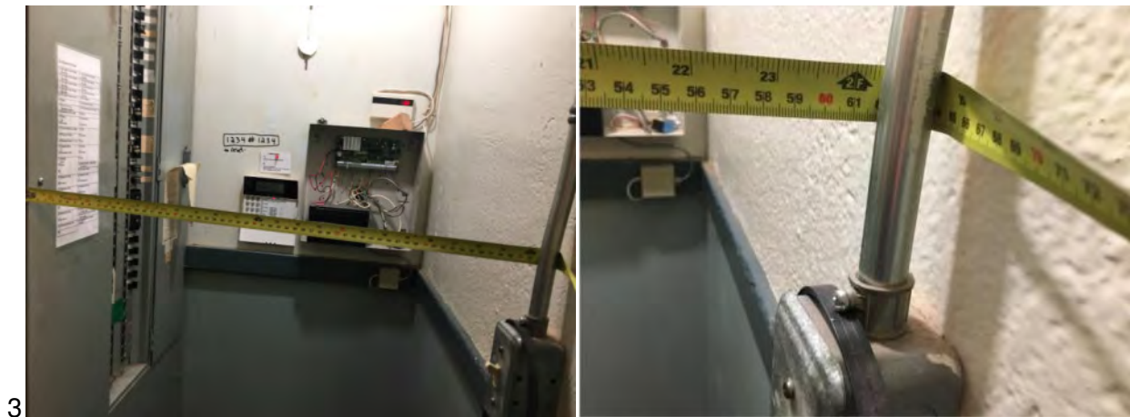
E12: Electrical Panel by ticket booth has less than one meter clearance
